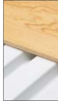
ROOF DECK WITH PLYWOOD FLOOR
