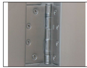
Fully Mortised Hinges (Shown on stainless steel door) Flush mortised hinges provide a clean and smooth finish to the door.
