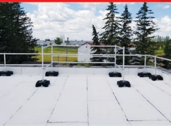
VSS Compact Guardrail and snow removal guardrail
